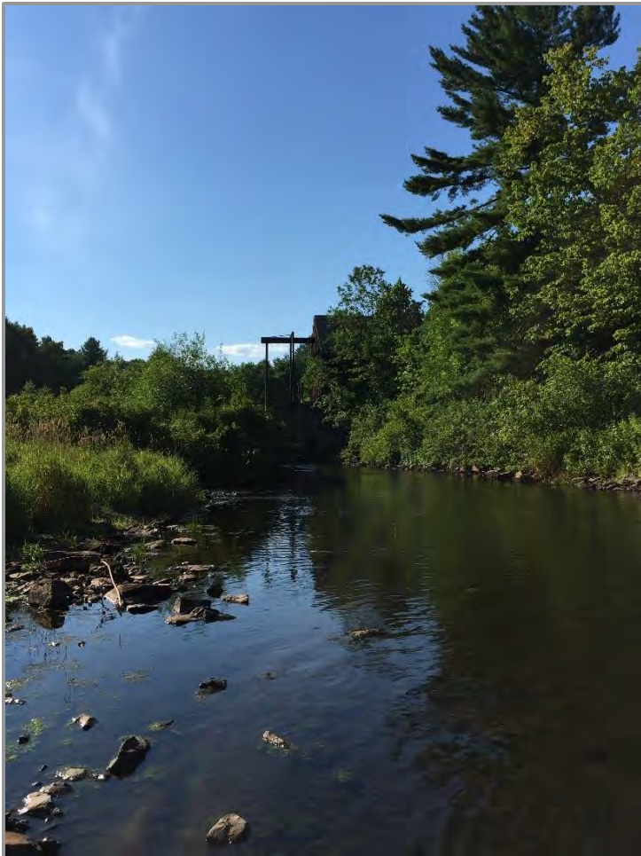
Photograph 8. (08/04/16) – View of non-tidal Cocheco Station 5 looking downstream (south).
